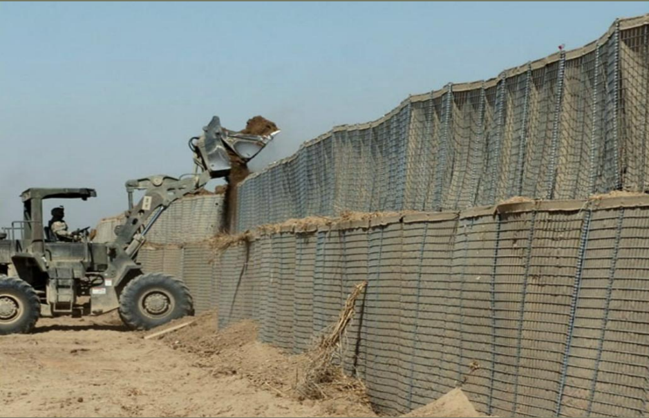
Construction of the Barrier
